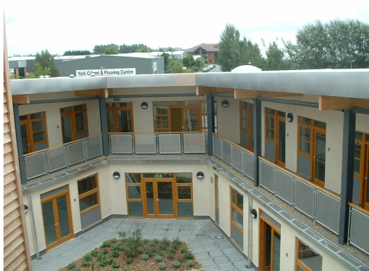
Eco Business centre Clifton Moor heated by Ground Source Heat Pumps.
