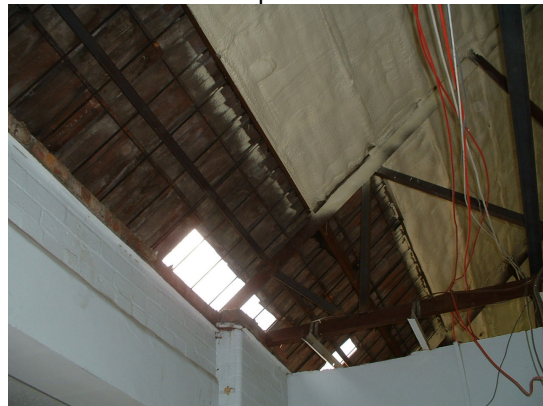
Improved roof insulation York High School (re-furbished from former Oaklands building)
